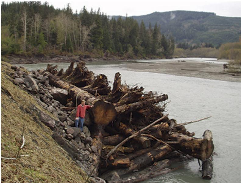
Figure 4. An example of a large engineered logjam built by the Washington State Department of Transportation on the bank of the Hoh River along U.S. Highway 101.
